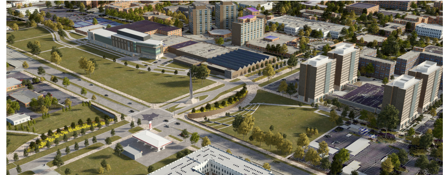
G2 3rd Street Tunnel & Entry Marker (Looking NE)
